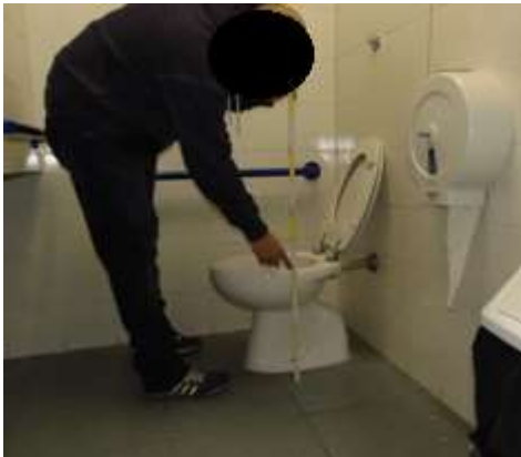
Photo showing the measuring of the height of the WC without the cover.
