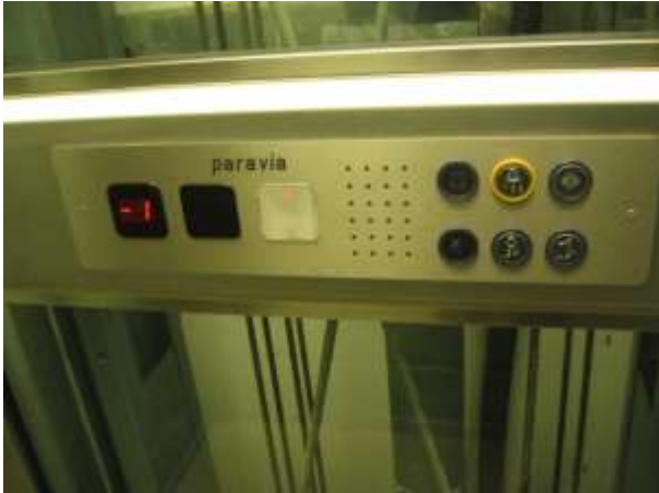
Photo of a button panel with light indications both embossed and in Braille.
