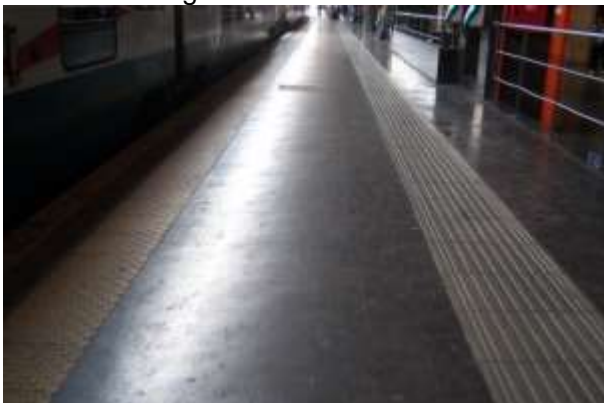
Photo of a train platform with two different tactile floor signaling. One is a strip on the ground near the external edge of the platform toward the rail. It is yellow and has embossed semispherical elements to warn of danger. The other is a light grey tactile path.
