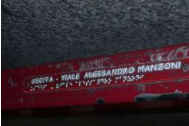
Photo of a tactile indication with colour contrast, embossed and Braille texts.
