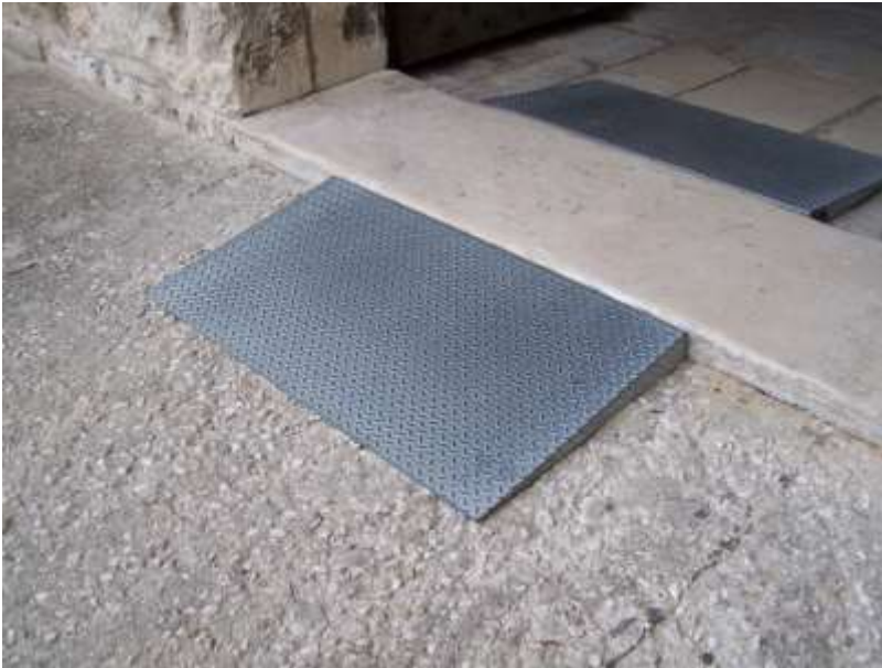
Photo of an external and internal threshold with removable ramps
