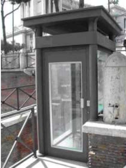
Photo of an elevator from outside
